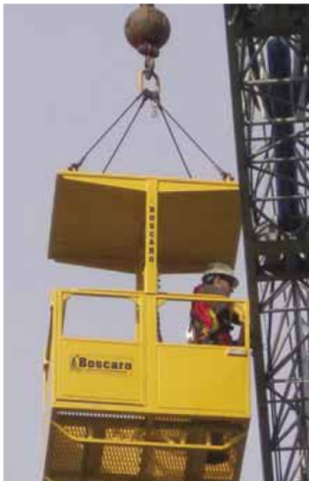
The Boscaro personnel basket has an access door and wraparound inner safety railing.
